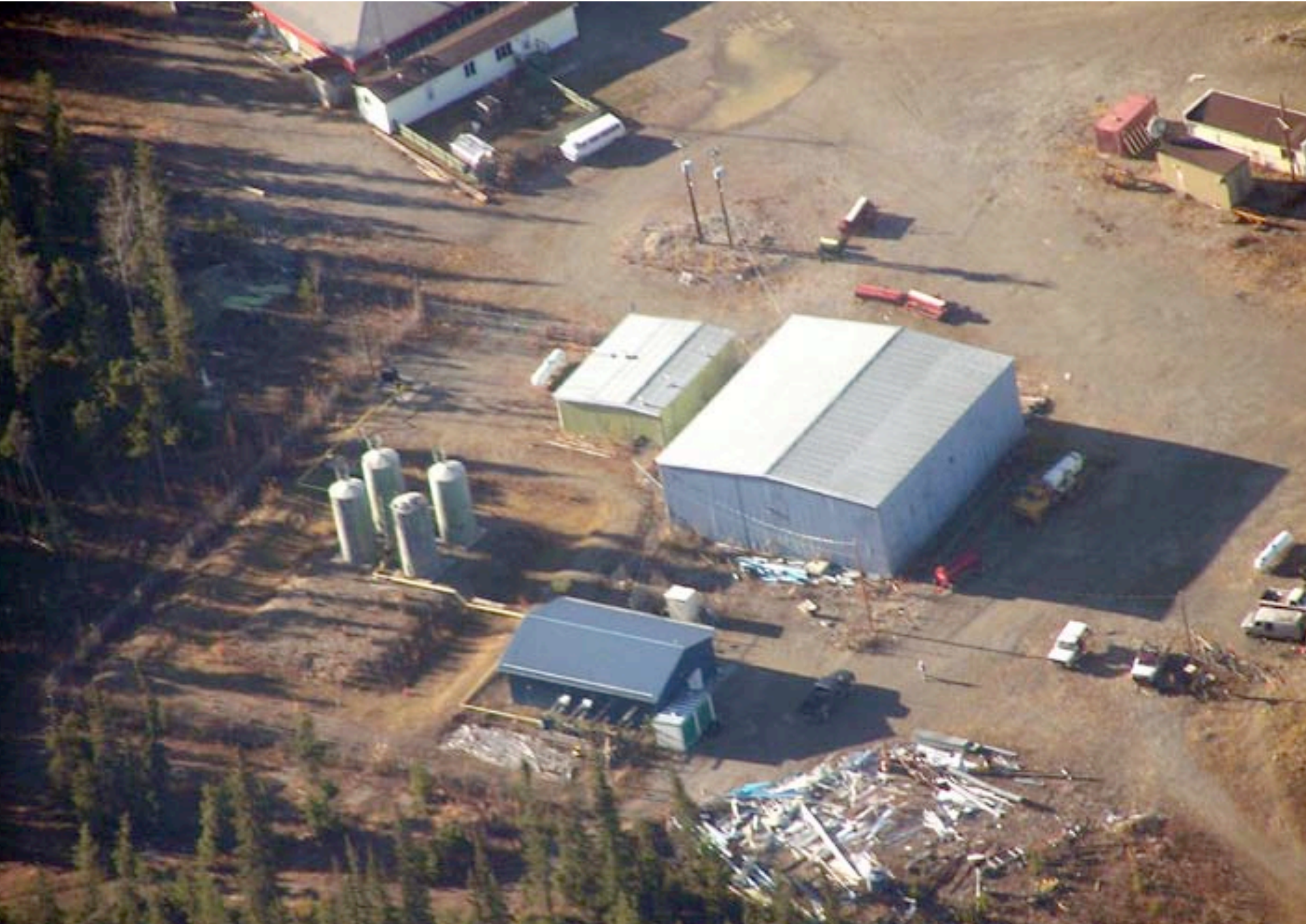
Generating Station in Tsay Key Dene
